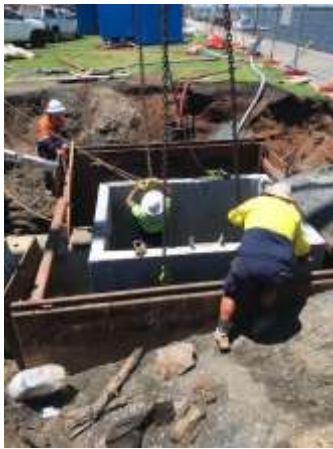
From left to right: installing pre-cast pit; installing the floodgate; the HDPE floodgate at the factory.
