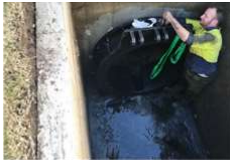
From left to right: installing pre-cast pit; installing the floodgate; the HDPE floodgate at the factory.
